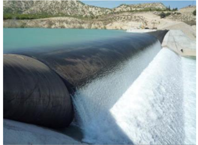
Fig. 9 Aquadam installed at Azmak Hydroelectric, Turkey
