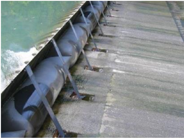
Fig. 8 Obermeyer Gates with a small flow overtopping
