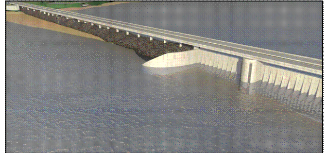
Fig. 13 Impression of a new crossing of the Solway Firth incorporating VETT units and a roadway. (Produced for Solway Energy Gateway Ltd.)
